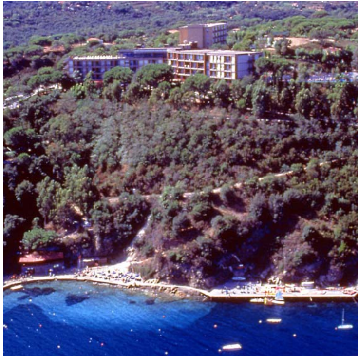
The splendid view enjoyed from the Hotel Elba International ****, a huge complex managed by the Apice systems designed using LonWorks and the Movicon Scada software.
