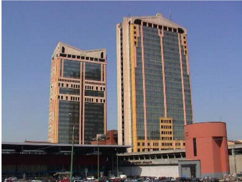
The Milan Porta Garibaldi railway station skyscrapers controlled by the PICodata bus and the Movicon supervisor.
